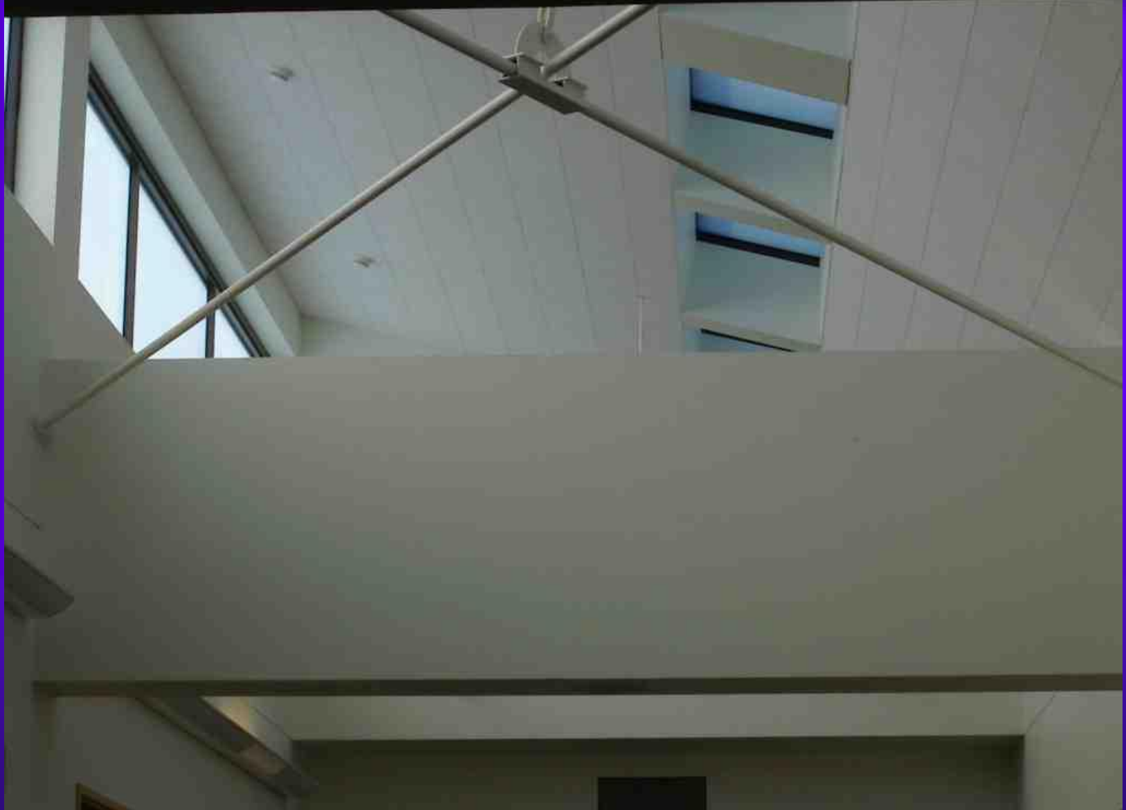
Horizontal and Vertical Hallway skylights
