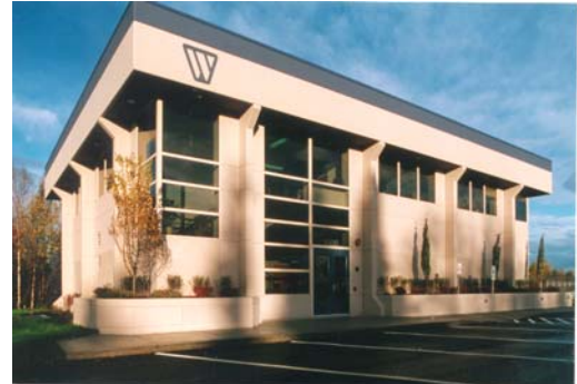
Watterson Construction Office Bldg. completed in 1999
