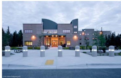
Barracks Complex @ Ft. Wainwright, AK
