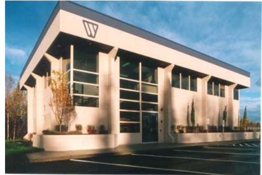
Watterson Construction Office Bldg. completed in 1999
