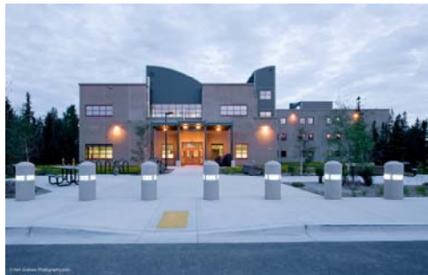
Barracks Complex @ Ft. Wainwright, AK
