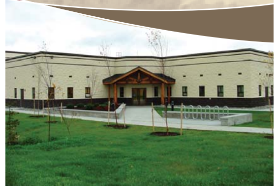
206th Combat Communication Facility Elmendorf Air Force Base, Anchorage, Alaska
