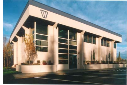
Watterson Construction Office Bldg. completed in 1999
