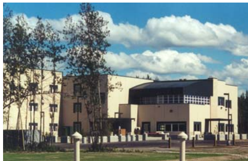
Barracks @ Ft. Wainwright, AK completed in 2000
