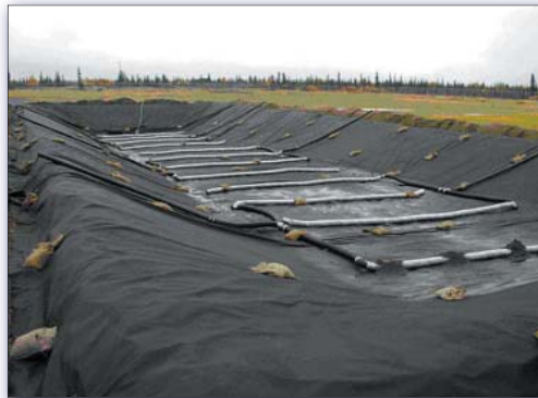
King Salmon biocell construction
